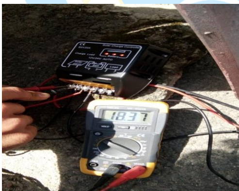
Gambar 13: Pengukuran solar panel
